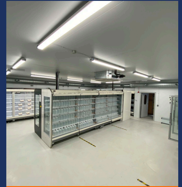
Refrigeration Research Centre
