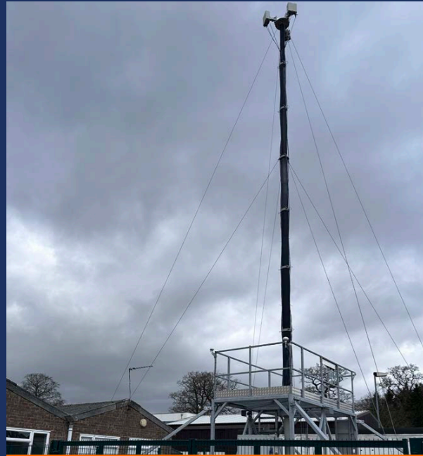
Mobile 5G-SA Mast
